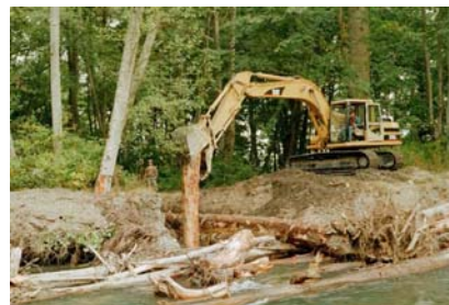
Installation of large woody debris.
